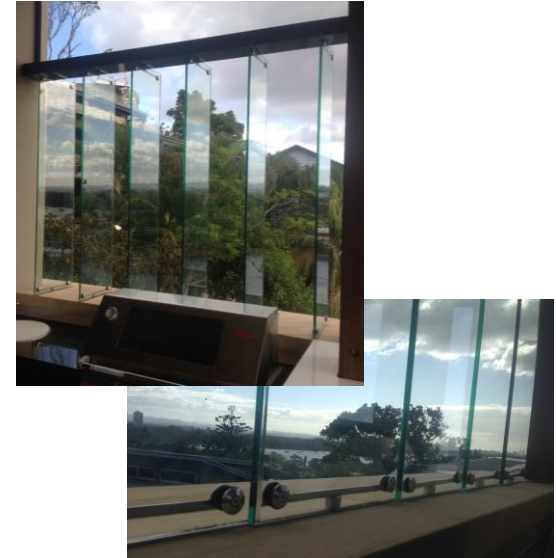
Vertical pivot glass louvres with concealed motor Sydney Residence
