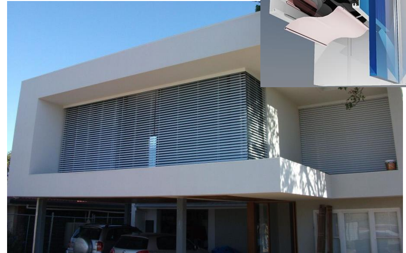
G.James / Liftmaster motorised external venetian blind integrated into window framing system.
