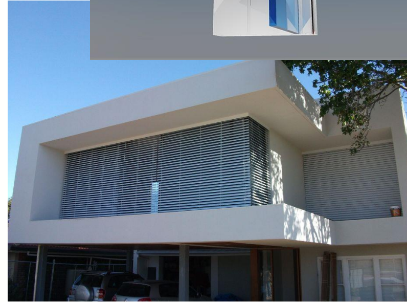
G.James / Liftmaster motorised external venetian blind integrated into window framing system.
