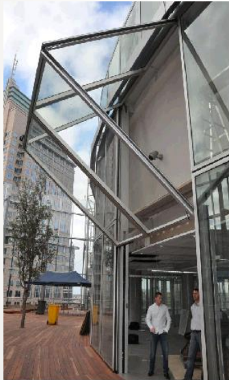
Vertical lift doors, No.1 Bligh St, Sydney
