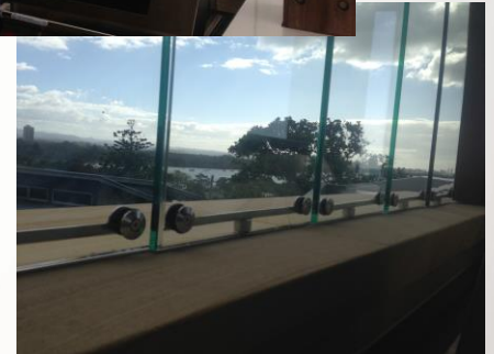
Vertical pivot glass louvres with concealed motor - Sydney residence
