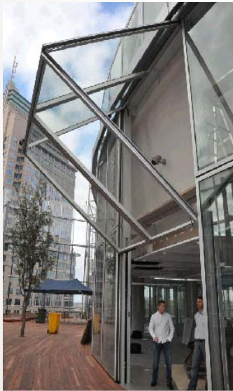
Vertical lift doors, No.1 Bligh St, Sydney
