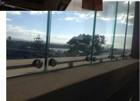
Vertical pivot glass louvres with concealed motor - Sydney residence
