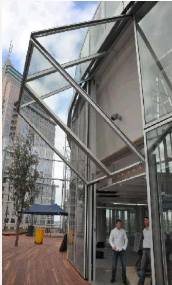
Vertical lift doors, No.1 Bligh St, Sydney
